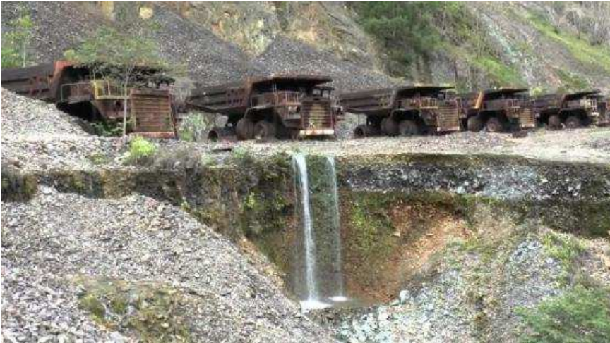
Rusting trucks at Panguna mine, Bougainville
